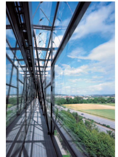
Double Facade as a thermal bufferzone and as an effective acoustic barrier to the autobahn
